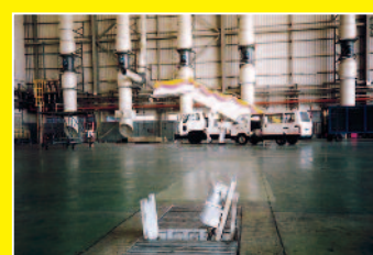
Aviation maintenance hangar
